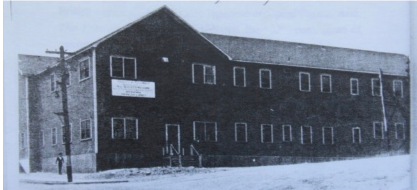
Knights of Columbus Hostel, erected December 1941
